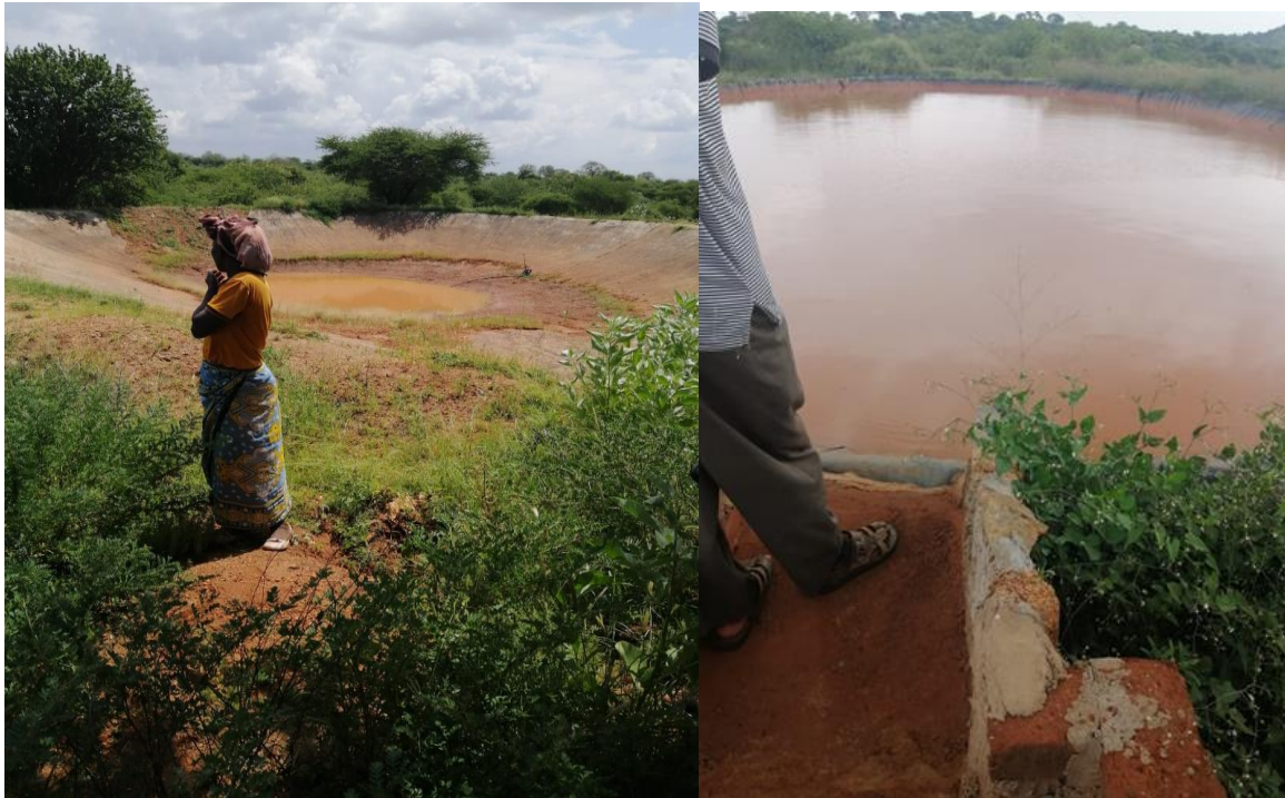
Figure 5: Earth Dam at Maragwa
